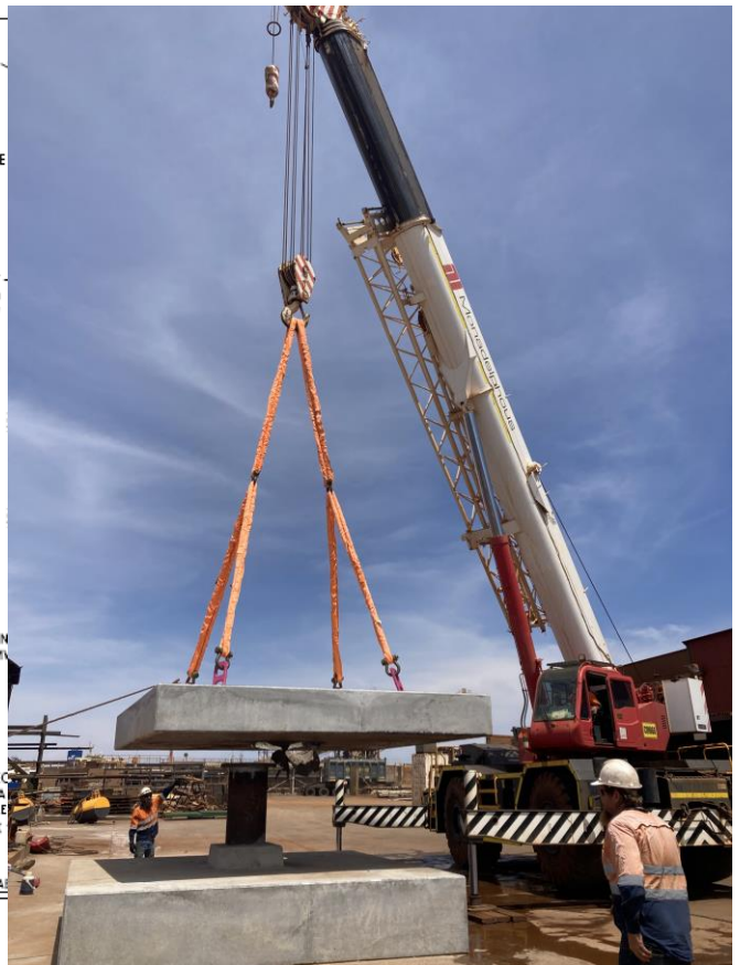
Lifting the precast base units
