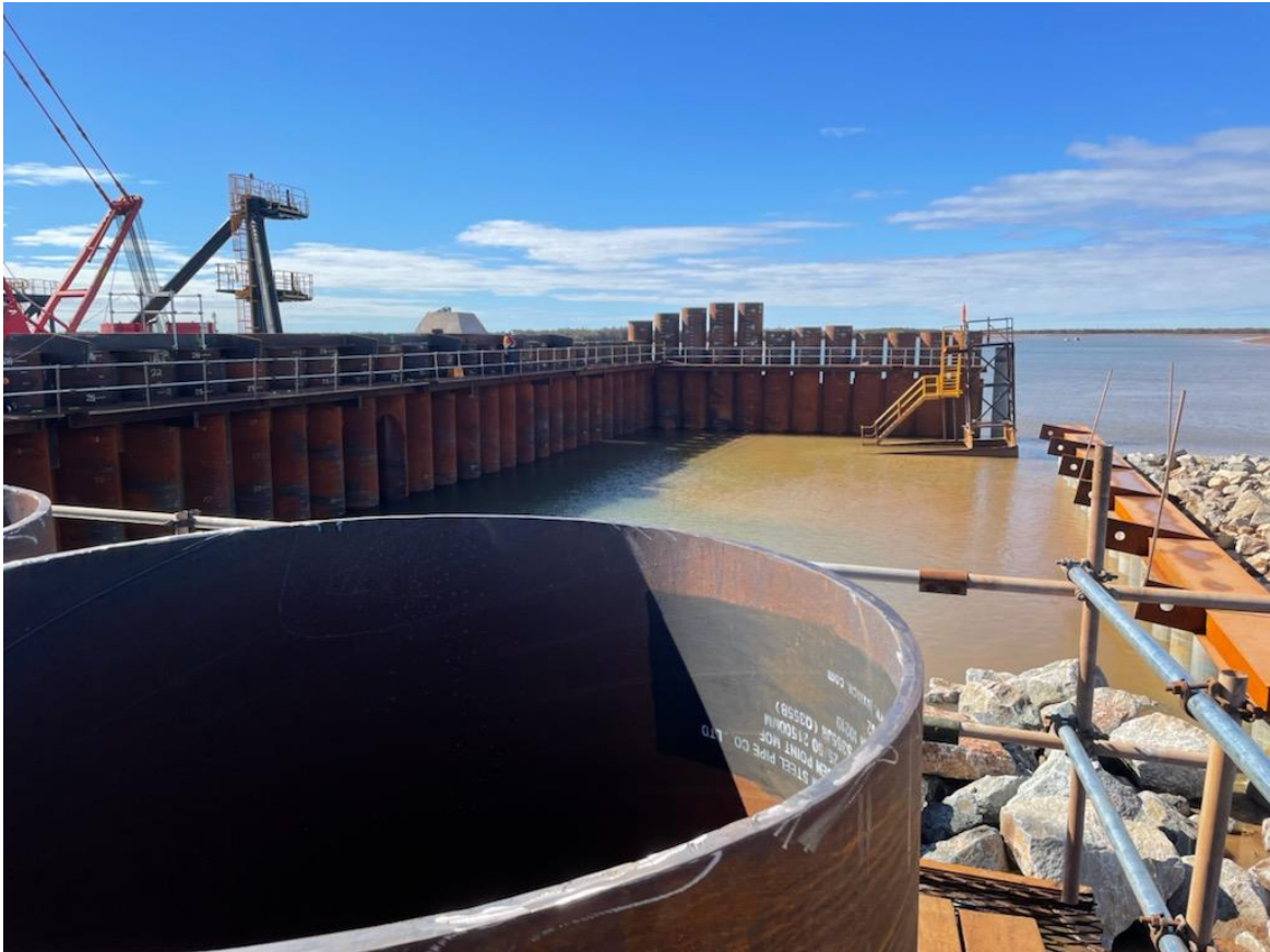
Backfilling behind the anchor wall + tie installation
