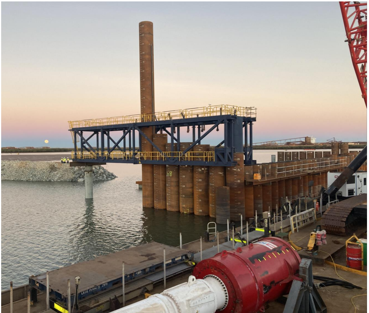
60t piling frame supported on temporary piles
