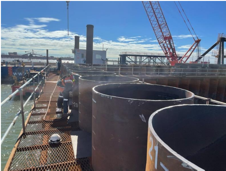
Access decks on main wall
