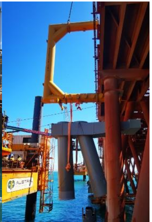
C Beam lifting 28t pile jacket under maintenance deck
