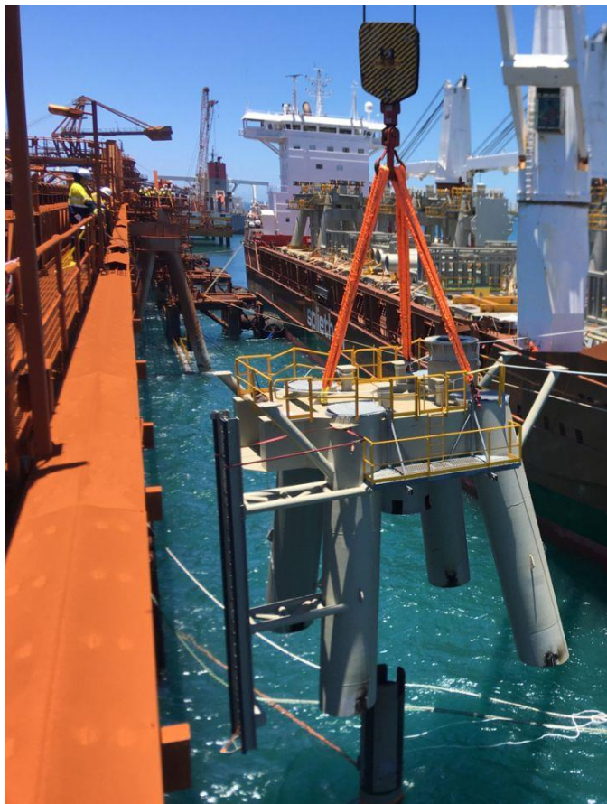
Jacket lift onto spud pile – max 120t
