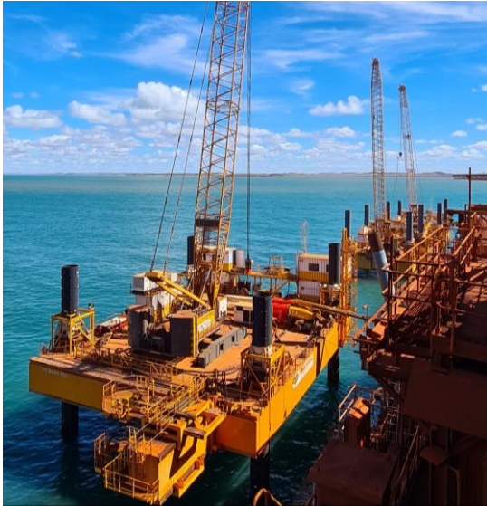
Three jackup barges working in the berth pocket
