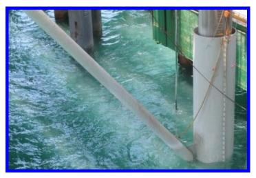
Roam Marine designed a grouted sleeve and brace to repair pile that was severely damaged by a tug at Cape Lambert wharf.
