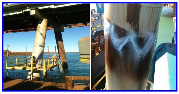
Roam Marine designed patches and sleeves to repair corroded piles on EII Jetty. Shown in picture is Roam Marine's "Horseshoe" 2 Level access platform used to weld on patch or sleeve and blast and paint.
