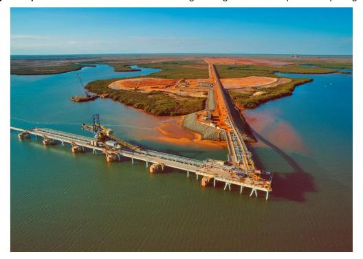
The review proposed changing the shiploader type which reduced the rail centres from 36.8m to 14m. This resulted in considerable savings in wharf structure, improved maintenance access and made it possible to modularise the wharf deck.
