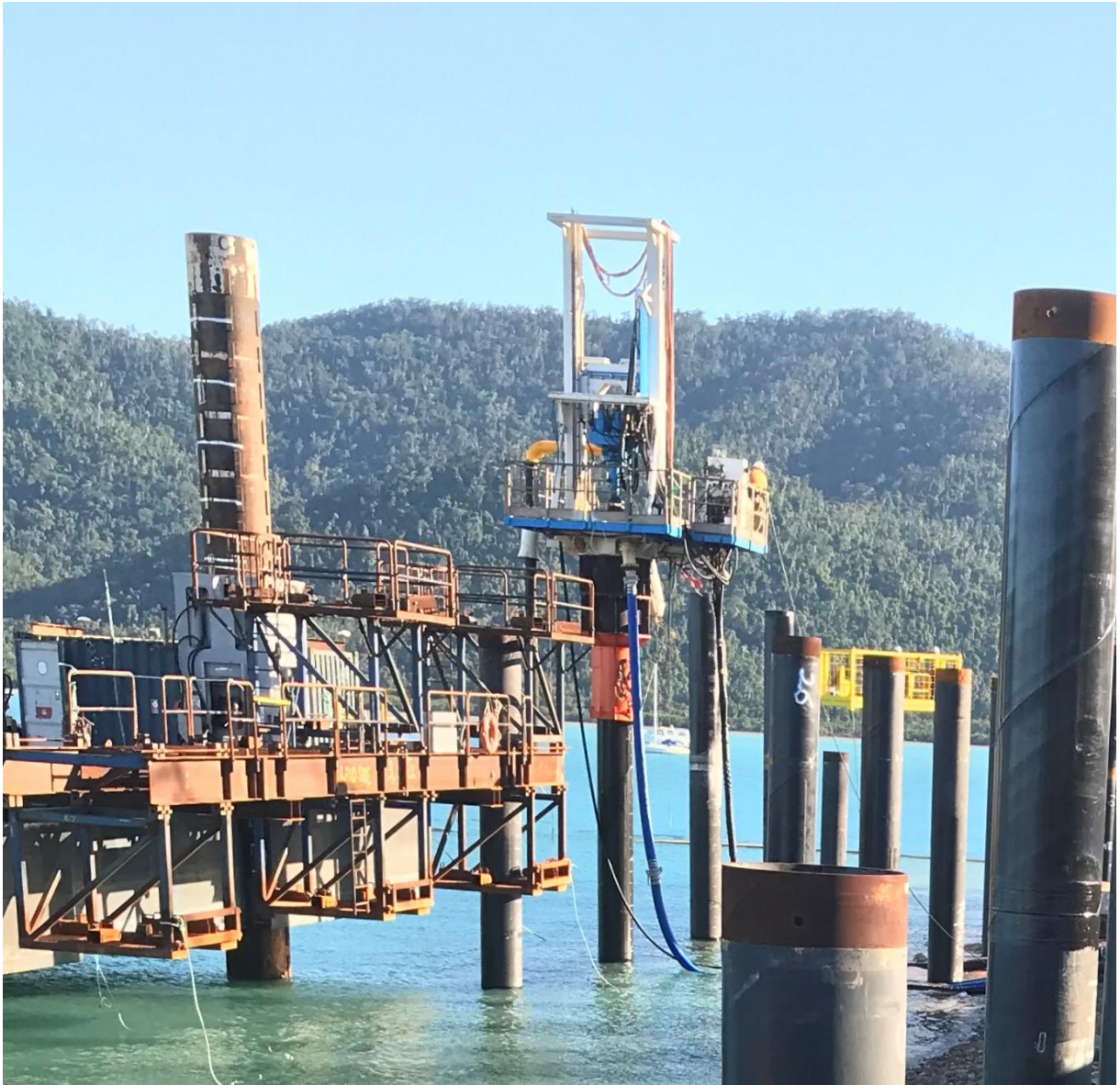
Piling gates and drill
