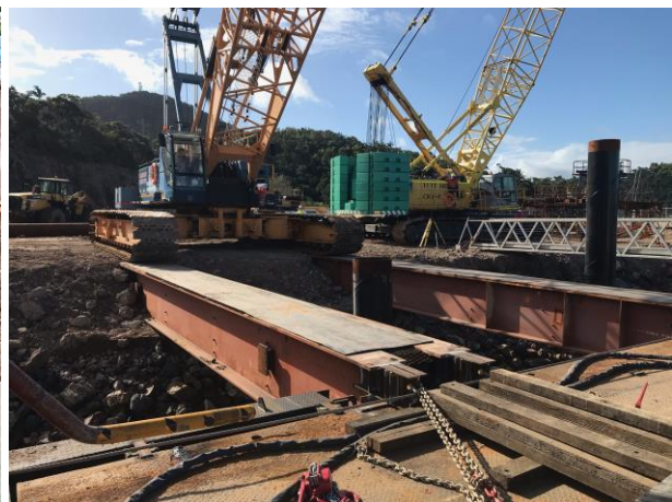
150t crane walking onto JUB
