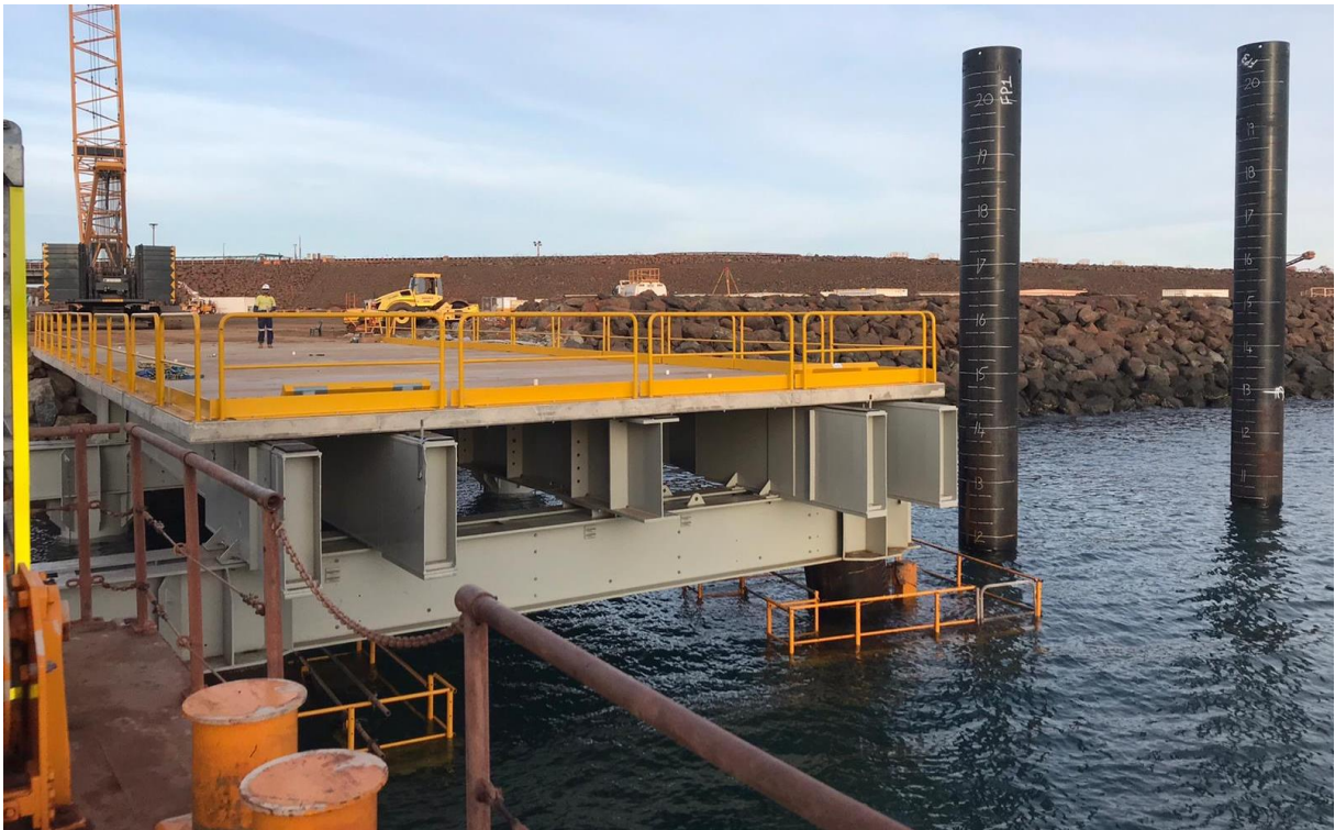
Jetty at high tide prior to pontoon installation
