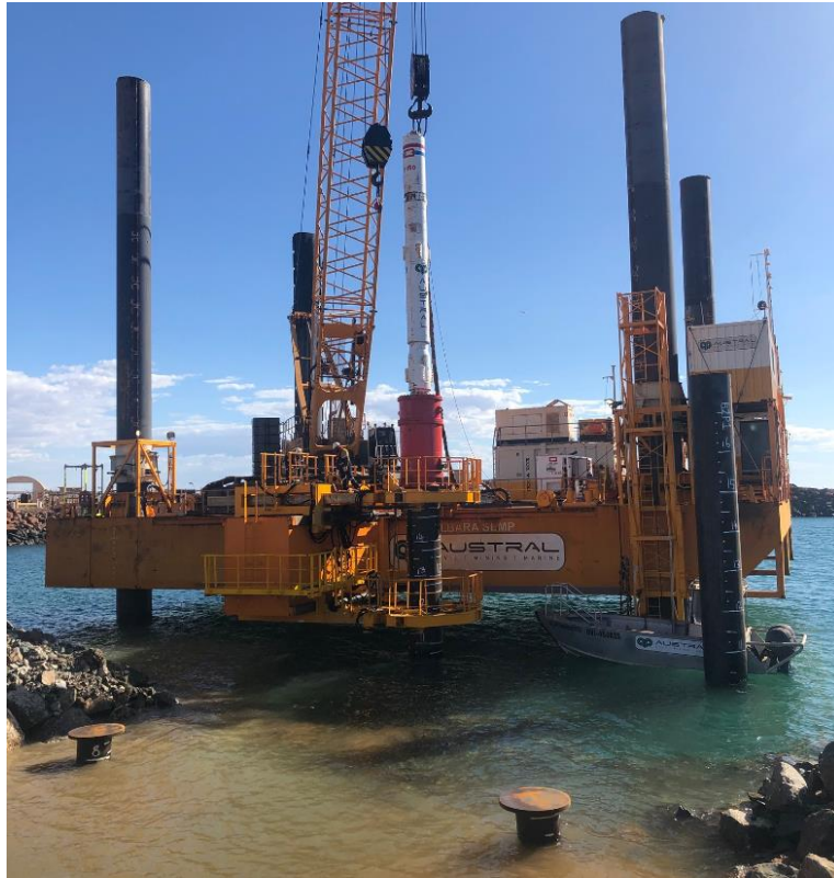
400t jackup with abutment piles in foreground
