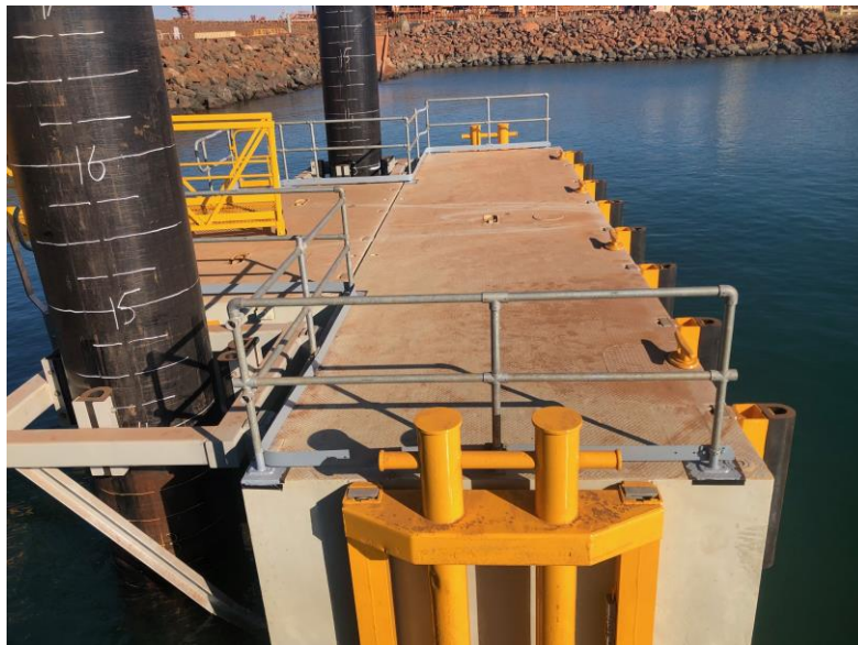
Pontoon with pile guides
