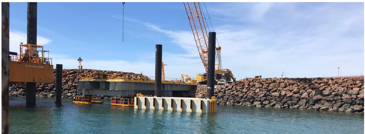
Berth 6 formwork, 40t pile caps and driving 2.2m 50t pile
