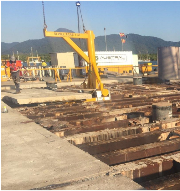
Berth Concrete deck removal
