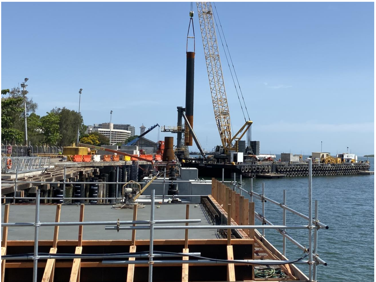
Berth 6 formwork, 40t pile caps and driving 2.2m 50t pile
