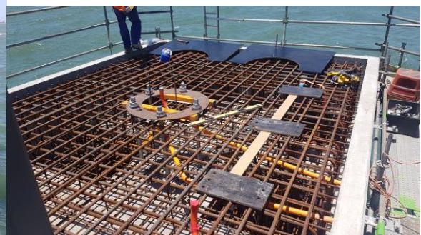
Precast dolphin shell
