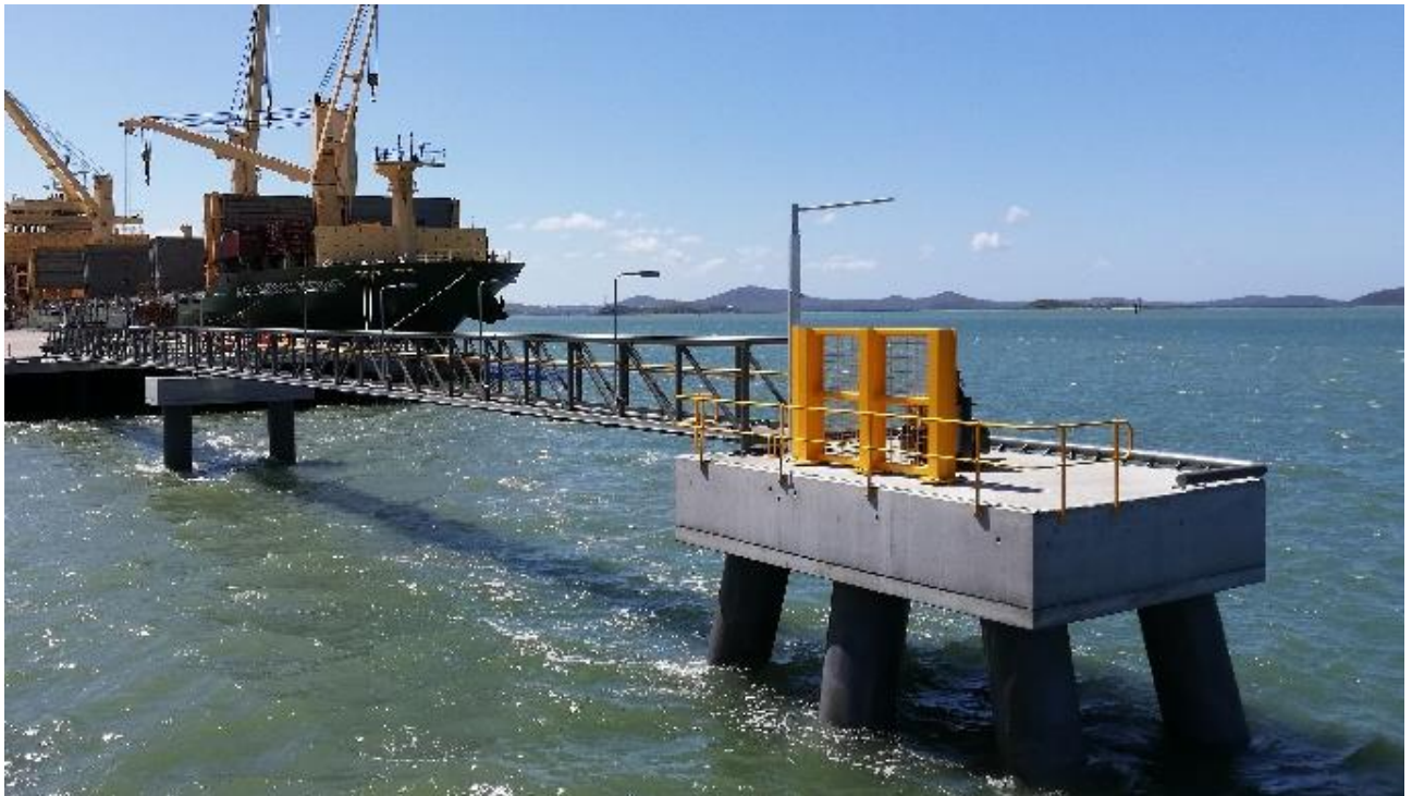
Dolphin and catwalks
