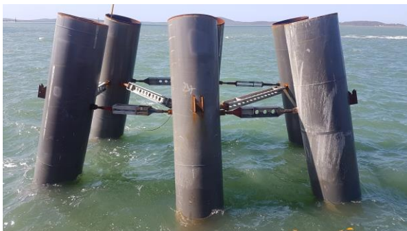
Pile bracing
