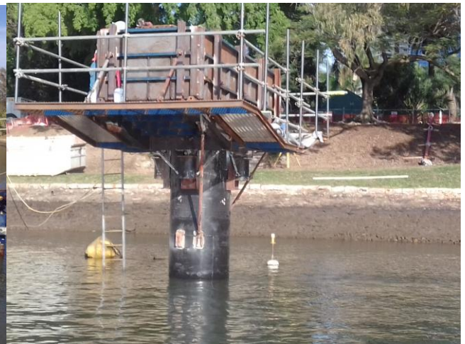
Pile cap form
