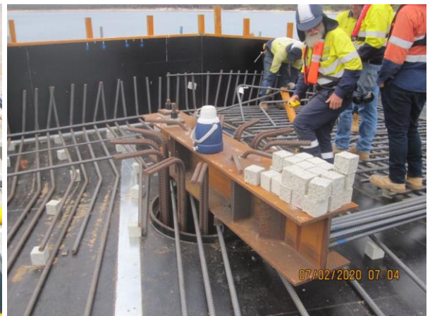
Pile cap and stress bars
