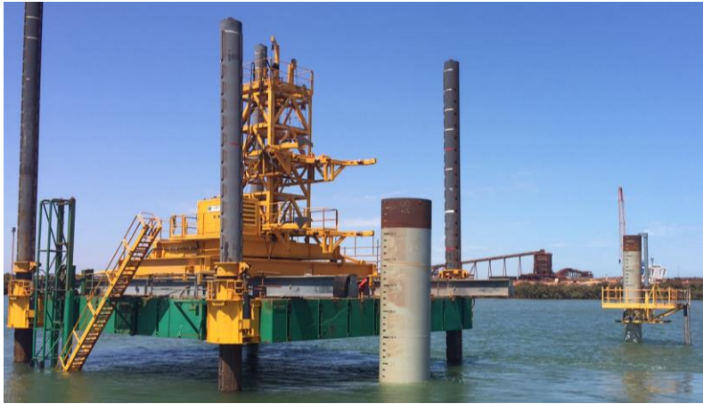
Existing pile frame mounted on jack-up barge to drive 2m diameter mono piles.
