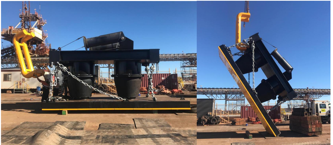
Installation of complete fender assembly with custom 25t C hook. Lift, rotate and install under edge of the wharf including scaffold access for brace installation.
