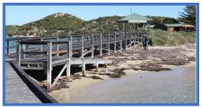
Existing Boardwalk had deteriorated due to material choice and harsh environment. Products chosen for the new boardwalk were to minimise maintenance. Combining FRP sections with Replas decking and stainless steel fixings throughout the deck should withstand years of use with no maintenance.
