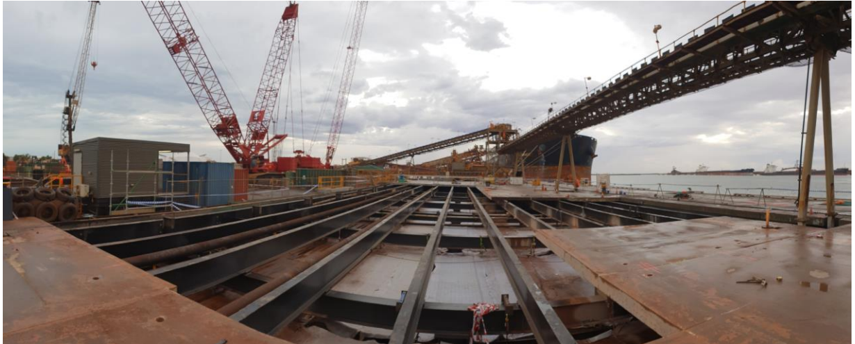
Suspended access and concrete cutting – note concrete lifts beneath overhead conveyor
