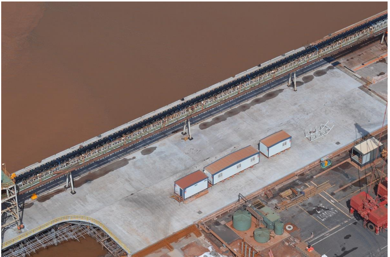
Third concrete pour 7 weeks after start of the shutdown
