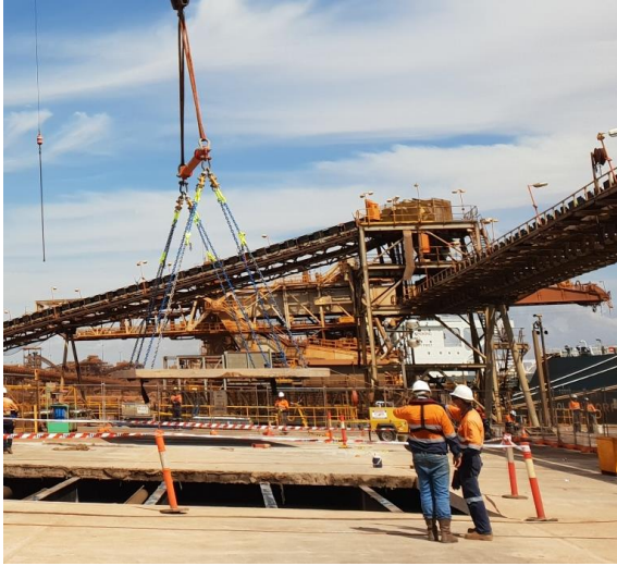
Concrete deck removal – up to 60t
