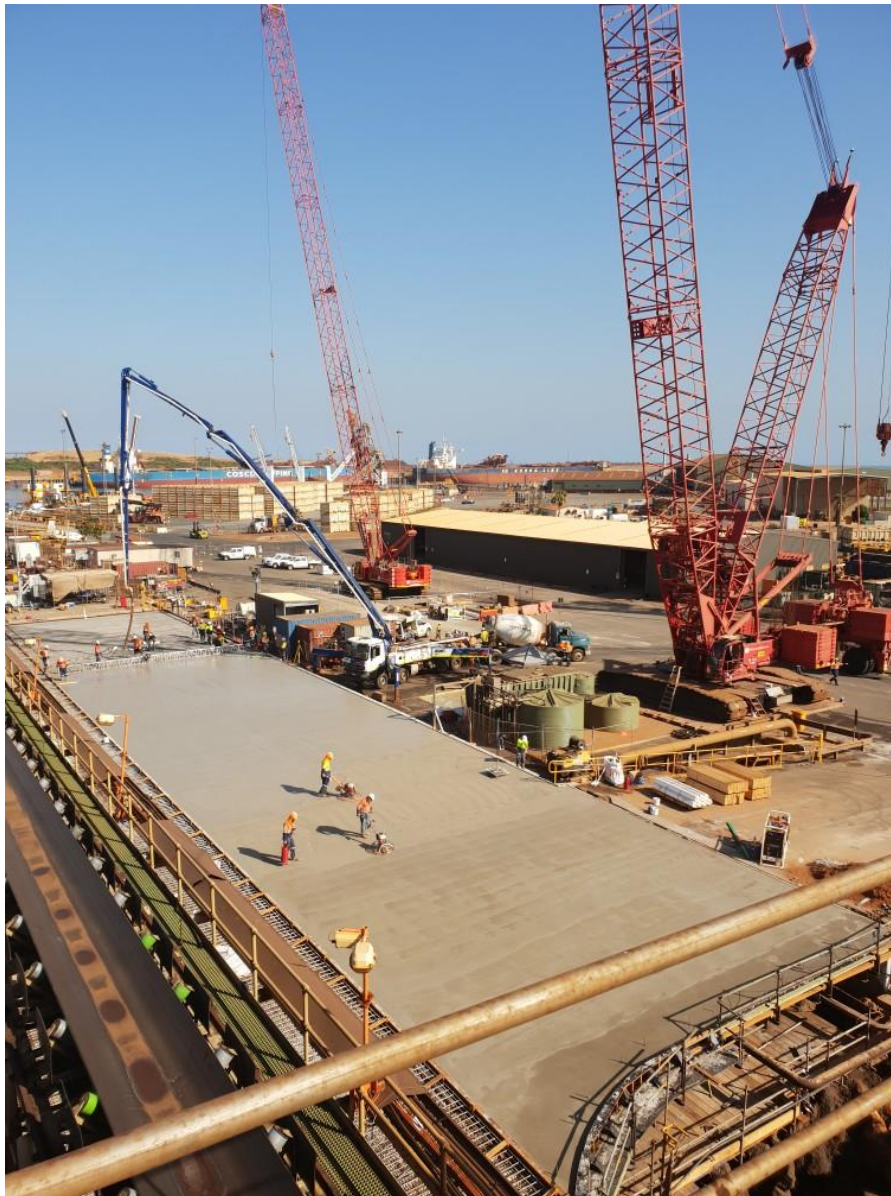
First concrete pour ~80m*15m was 5 weeks after start of the shutdown
