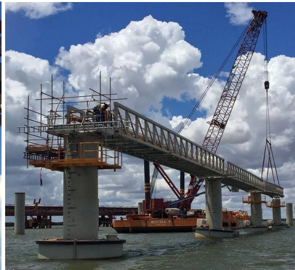
Walkway being installed
