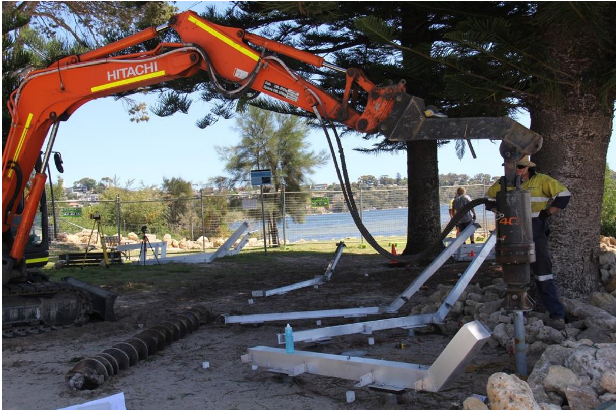
Installing the hidden structure at Pt Walter, Bicton
