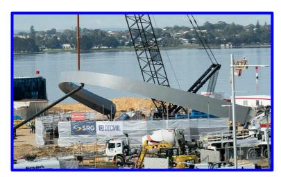
The walkway bridge is held up via 2 42t steel arches 17m tall and spanning over 32m onto the concrete piers. Each arch leans over approximately 65 degrees. The lift was intricate involving a sliding central prop and rotating base. The arch rotates from horizontal up and into position then site welded to the baseplate which is attached to the concrete pier via macalloy hold down bolts. Roam Marine did full verification on lift design.
