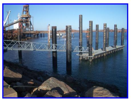
included scope power, lighting, cathodic protection and water services. The mooring piles were fitted with 200t breaking load vertical cables 8m long with heavy lugs welded to the piles. Tugs can safely cyclonic moor in conditions and handle a 9.5m storm tide range.
