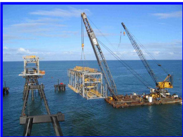
Lifting and placing Section2 and the 102t shuttle that slides inside the main box truss on rollers
