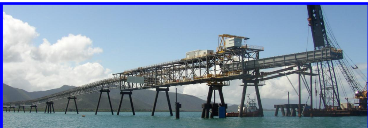
Lifting and placing Section2 and the 102t shuttle that slides inside the main box truss on rollers
