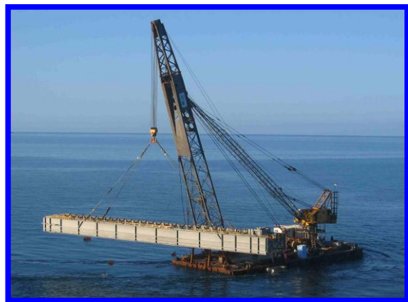
Lifting and placing Section2 and the 102t shuttle that slides inside the main box truss on rollers
